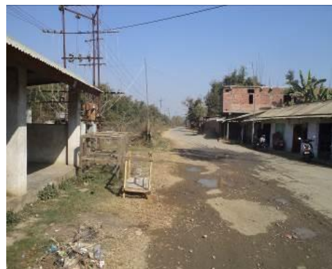
Potholes due to lack of Drainage Facilities
