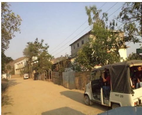
Road Condition near Shija Hospital
